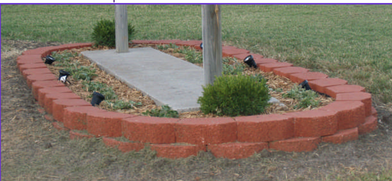
Landscaping work around the base of the new church sign
